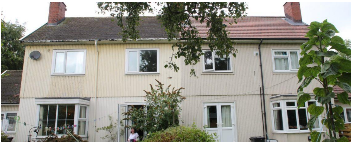
Swedish Houses Type A, rear view, Pool-in-Wharfedale (Prefab Museum)
